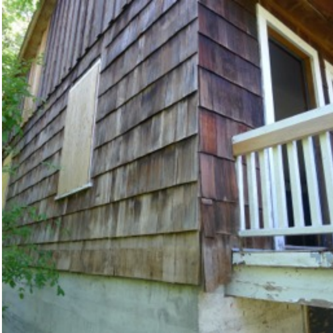
West side of the house showing the original window pattern, shingles and board and batten siding including the new material in the gable to match the existing siding pattern
