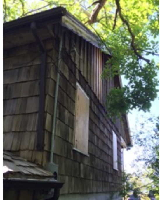
West side of the house showing the original window pattern, shingles and board and batten siding including the new material in the gable to match the existing siding pattern
