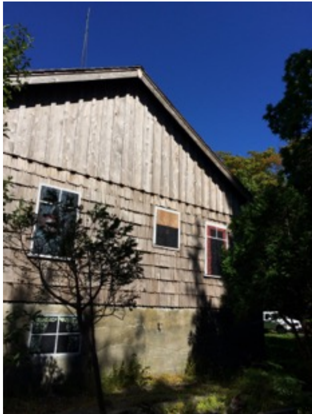
East side of the house showing the shingles and board and batten siding and original window positions.
