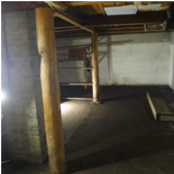
Above: The basement features logs as posts supporting the main floor of the house
