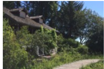
The house from the footpath and boardwalk
