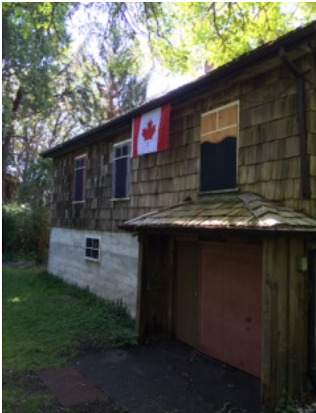
Rear of the house showing the shingles and original window pattern. The roofed entrance to the basement is on the west side of the rear. From this position the high basement foundation is most prominent
