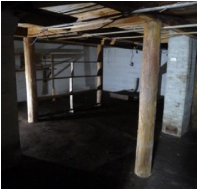
Above: The basement features logs as posts supporting the main floor of the house
