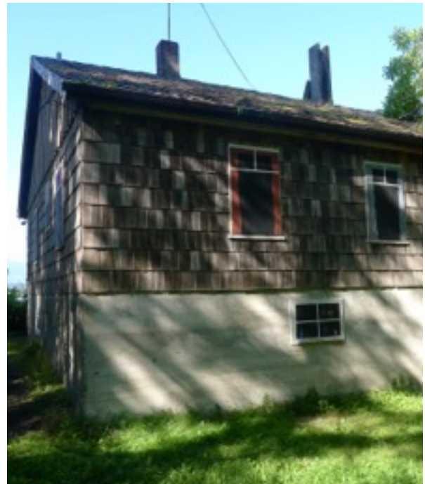
Rear of the house showing the shingles and original window pattern. The roofed entrance to the basement is on the west side of the rear. From this position the high basement foundation is most prominent
