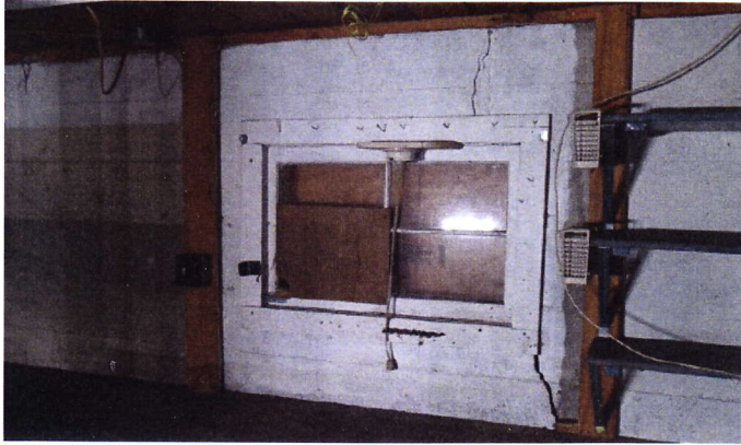
The cracks in the foundation. Inside south wall, exterior north wall
