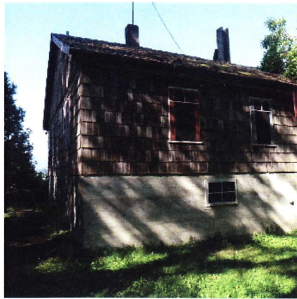
High concrete foundation
