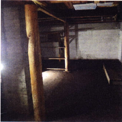
Basement with log posts and platform for washer and dryer.
